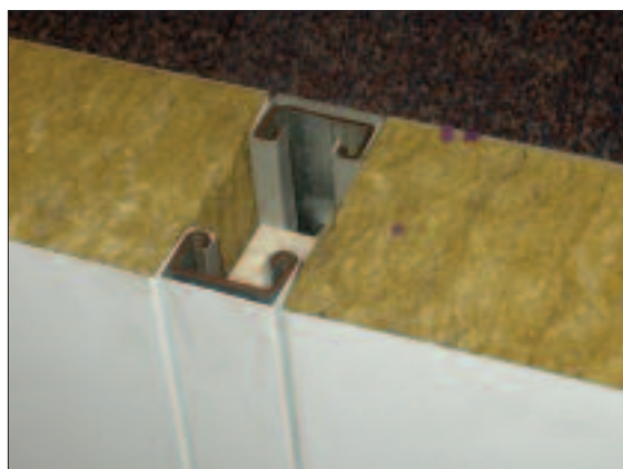
Figure 17: Insulated core panels – internal panel
