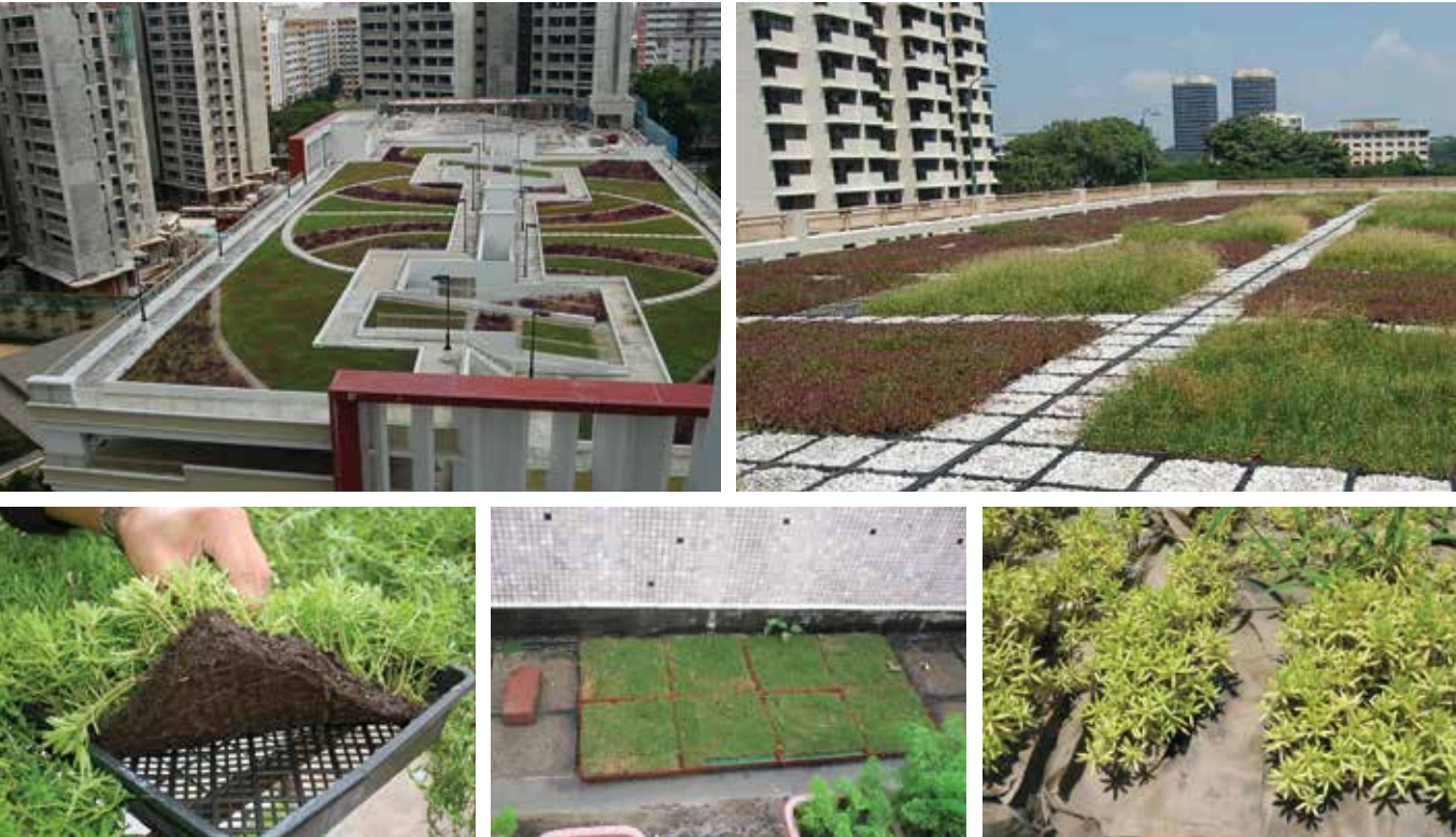
Figure 2.6 (bottom) Examples of modular green roof systems Left: Vegetated mat system Centre: Tray system Right: Sack system
