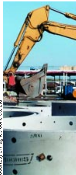
Precast concrete soakaway rings being installed for drainage of a supermarket car park
